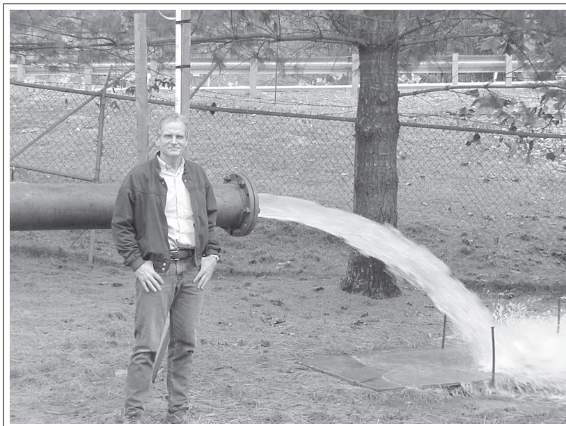
John Davis, Loudon Utilities Environmental Engineer, worked with Bradfield Environmental Services, Inc. to drill a total of ten wells, of which three produced substantial quantities of ground water.
